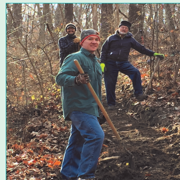
ORLT Stewardship Specialist Nic Rogers, ORLT Board member David Taylor, and volunteer Gary Schneider level and install water bars on a sloping section of the trail.
